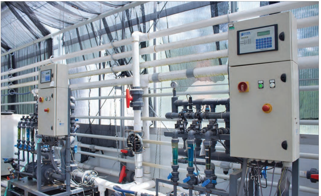
Two panel mount units used in a fertigation system
